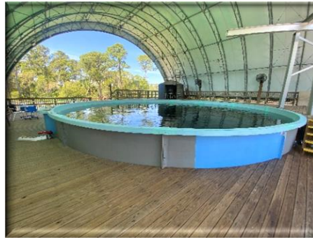
Figure 28: Stranding Station Pool COMMENT: Algae growth requires scrubbing.
