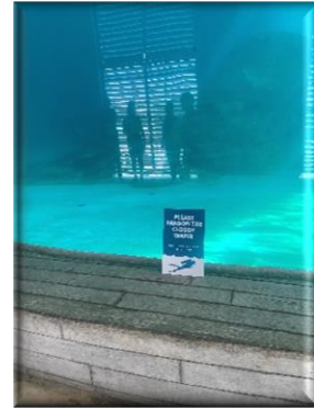
Figure 13: Algae Cleaning Causes Short-term Turbidity in Tank 5. COMMENT: Algae growth in system driven by direct sunlight from windows. Cleaning issues.
