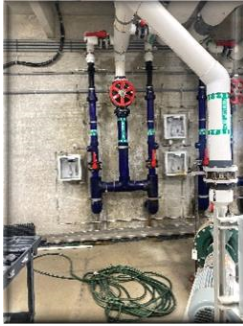
Figure 17: Ozone Injectors. COMMENT: Ozone injection used to control coliforms to zero. Consider reducing dosage to increase biological diversity
