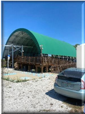
Figure 27: Stranding Station Facility
